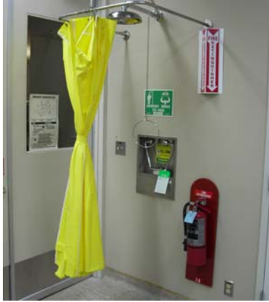
Safety shower, eye wash, and other safety apparatus in SNF
