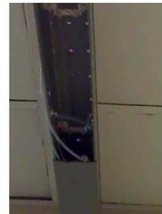
5. In addition to disconnected sample lines in at least one location the sample line has been cut and attached to another location. The photo below shows the back and top of the Thermco 2. The sample line to the gas jungle was cut and reconnected to the adjoining gas box. This has left the furnace unprotected. This furnace has Silane, Dichlorosilane, Diborane, and Phosphine which all need monitoring by TGO code.
